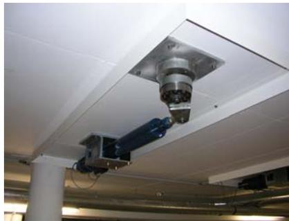
The thrust tube of the actuator is connected to the lever arm of the revolving glass door panel
