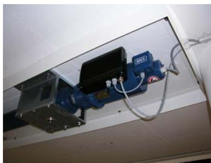
On board control via a variable frequency drive, position monitoring and end of stroke supervision
