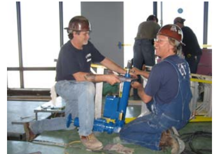
Mounting the Front Flange to the Actuator
