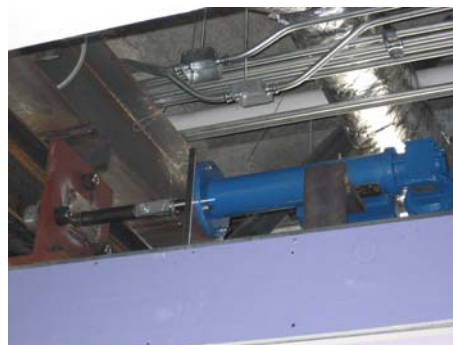
Locking Pin Actuator Securing the Ledge
