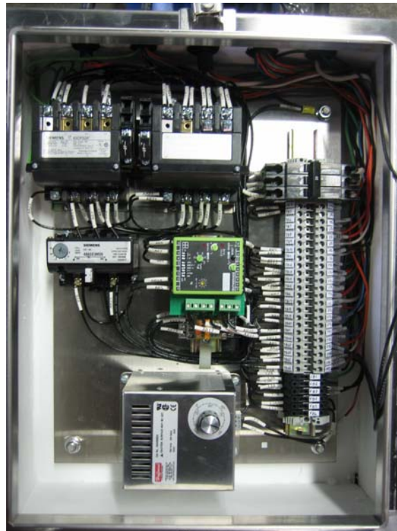
Heated Control Panel
