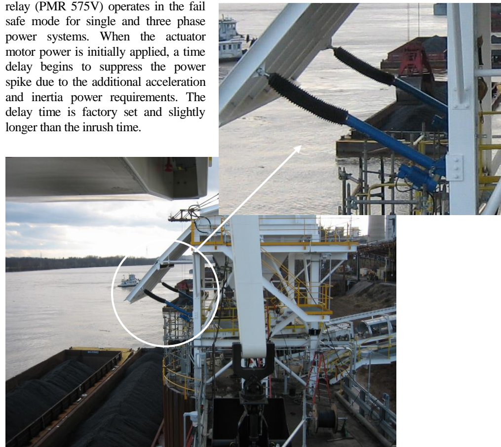
Coal Unloading Facility
