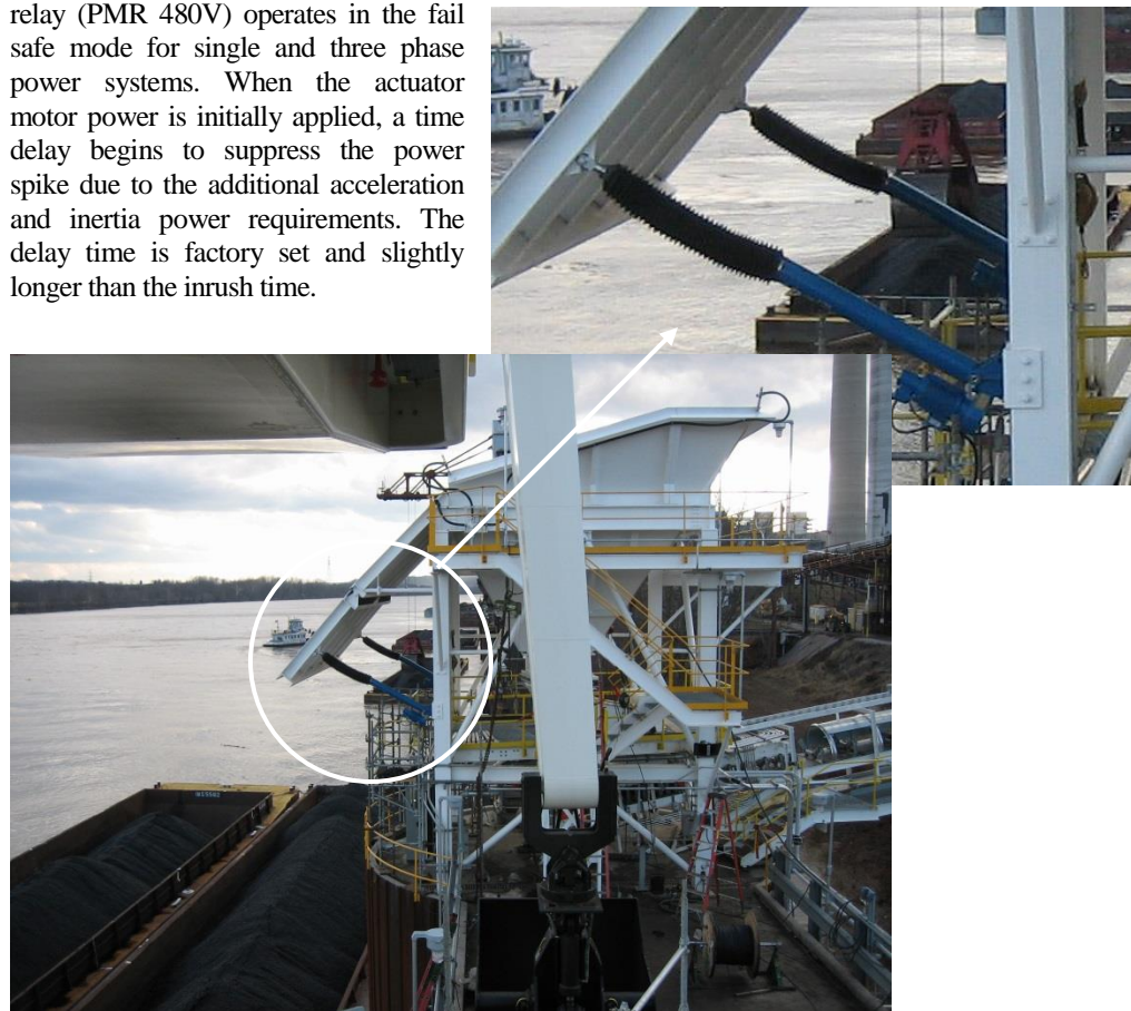
Coal Unloading Facility
